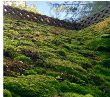
Top left to bottom right: Delicate native moss covers the pitched roof of this outdoor pavillion / Fireplace House roof blends into the lakefront hillside / Five different species of moss were planted into the roof
