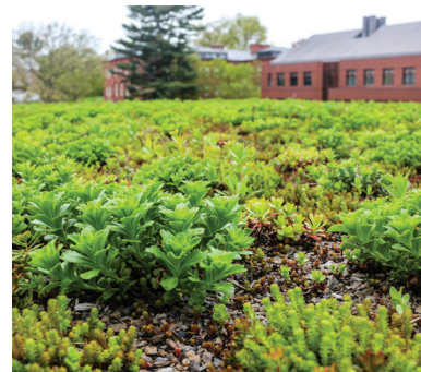
Top left to bottom right: Green roof is visually accessible from classrooms and offices in building/ Edging required painstaking detailing to match interior stone scape/ Many varieties of sedum were planted to provide visual interest throughout seasons.
