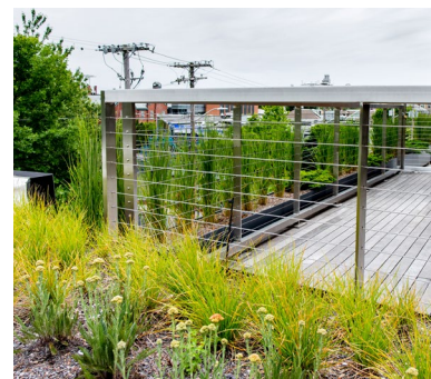
Top left to bottom right: A section of full-grown extensive trays with heuchera and Penn. sedge || Extensive trays immediately after planting || Edge of meadow and roof deck meeting the east parapet planters
