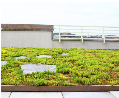
Top left to bottom right: A planter wall with perennial grasses creates a privacy screen between the sedum and lawn spaces / Gardening with a view in this corner raised bed / Mahogany trim caps separate the sedum and patio
