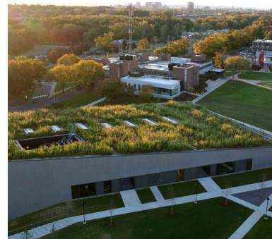
Top left to bottom right: The upward slope of the Hursey Center / Skylights and roof access points sunk into the living meadow system / The Hursey Center as a new centerpiece for the University campus
