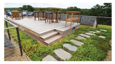
A peaceful green roof of sedum and hardwood decking sits atop this Vineyard home, which is located on a peninsula between two branches of a brackish pond. The roof adds a sunlit retreat to the building's living space, in addition to absorbing and slowing rainwater over its footprint.
