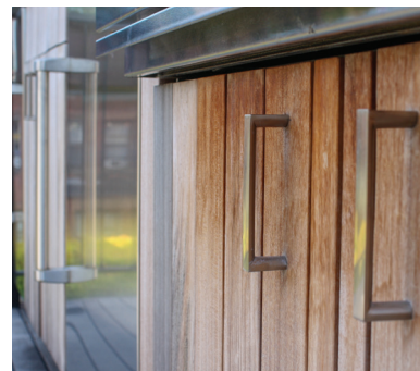
Top left to bottom right: Homeowners can enjoy dinner and a view from their custom summer kitchen / Sedum seed heads add texture at the edge of this roof deck / Recover installed custom stainless cabinetry and FSC-certified ipe cladding
